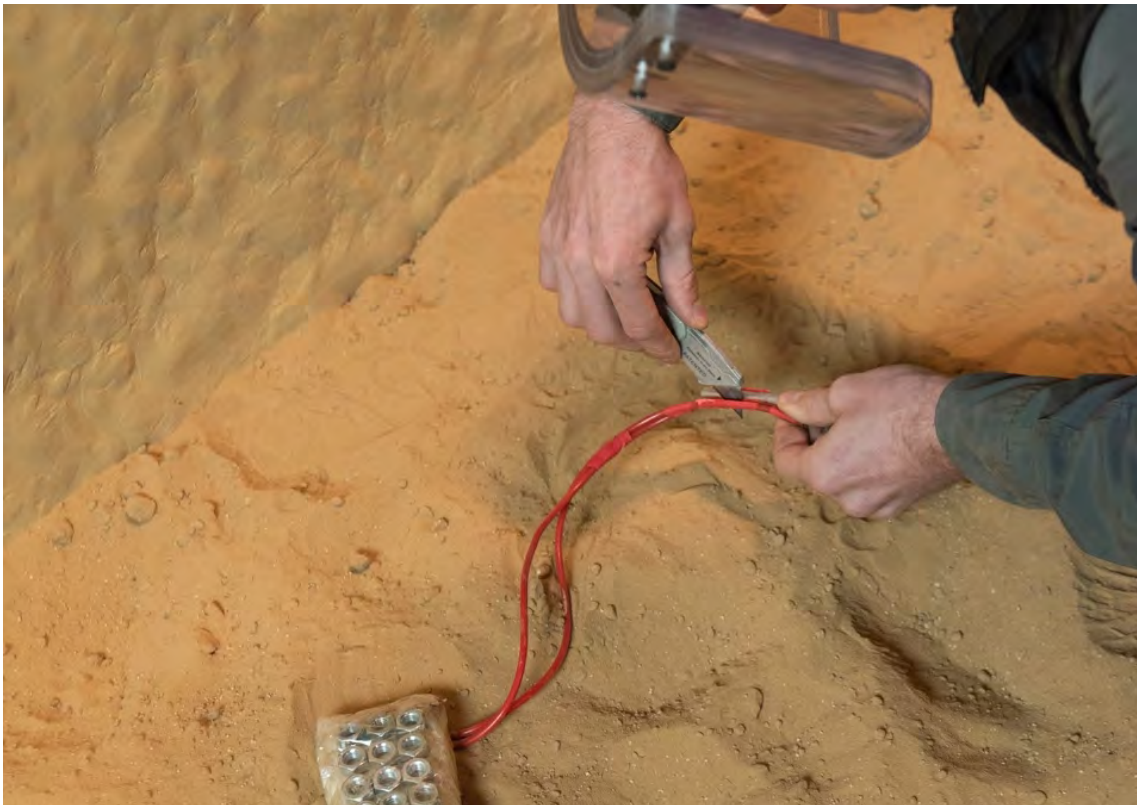
Image 5. Detonator is rolled slightly to expose the PAT on the other side. This is then cut in the same manner as above
