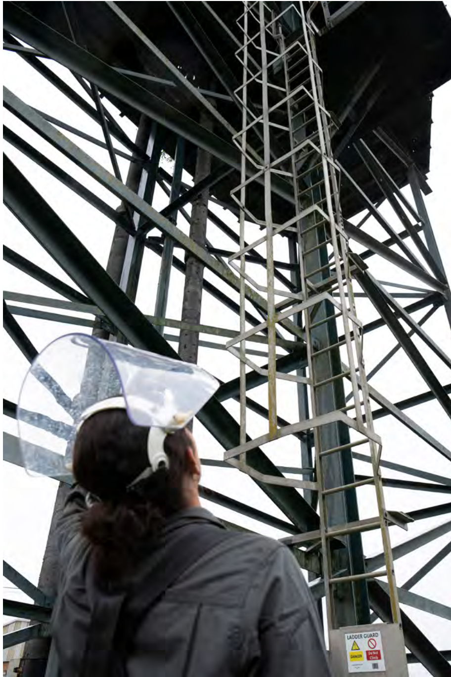
Image 8. A member of MA staff identifying a working at height hazard
