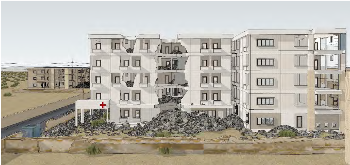
Image 1. Overview of the damage and debris preventing ROV access to the hospital
