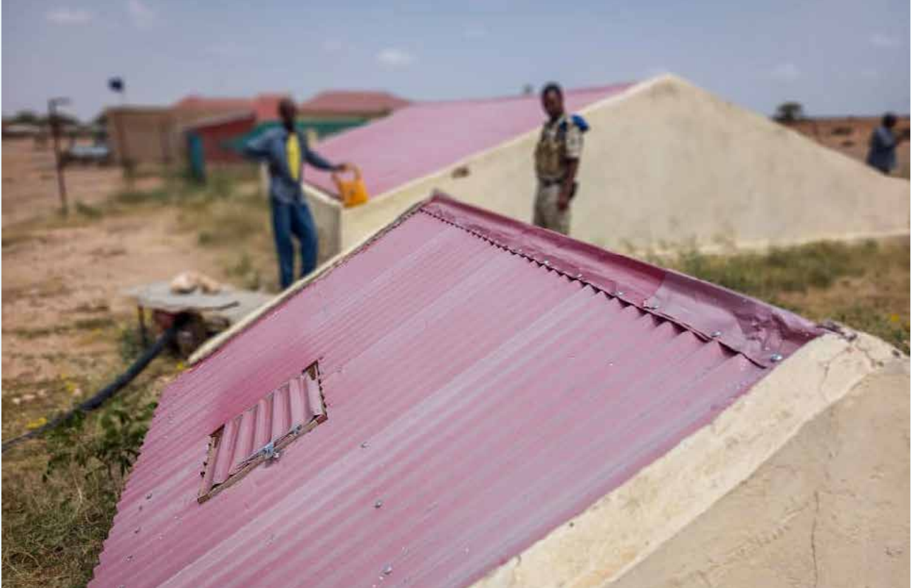
Community berkards constitute important water capture and storage structures, ensuring water availability in local communities. In Sayla Bari, Somaliland, mine action played a crucial role in facilitating the delivery of water to communities through the clearance of roads. This continues to be of critical importance in 2023, after six years of drought in the region. ©GICHD
