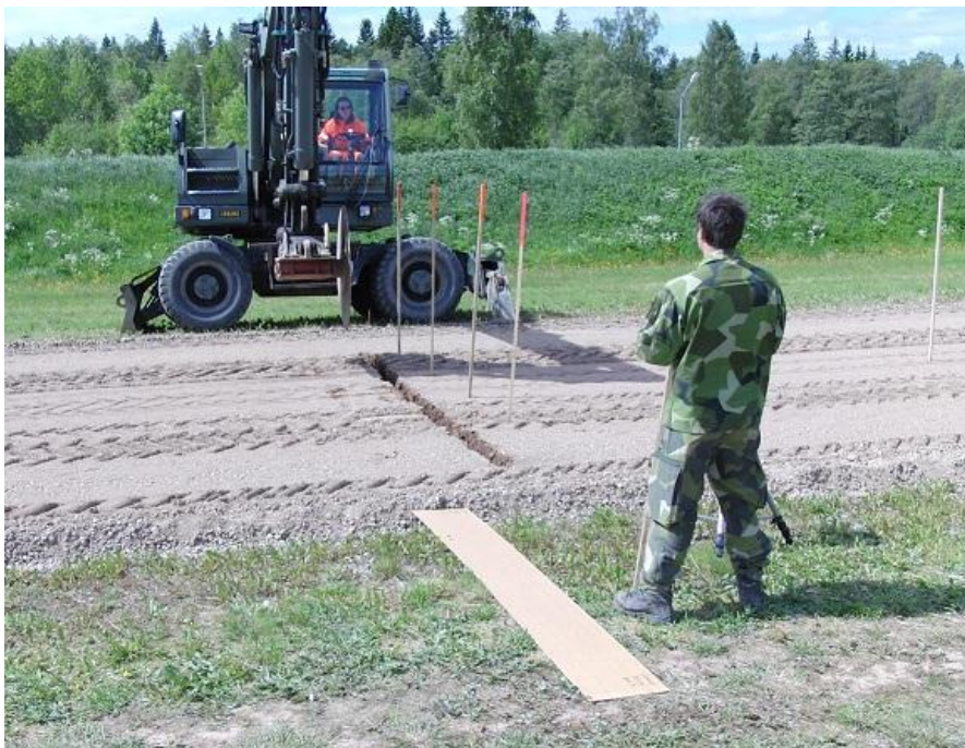
Figure 59. Preparing for planting a witness board.
