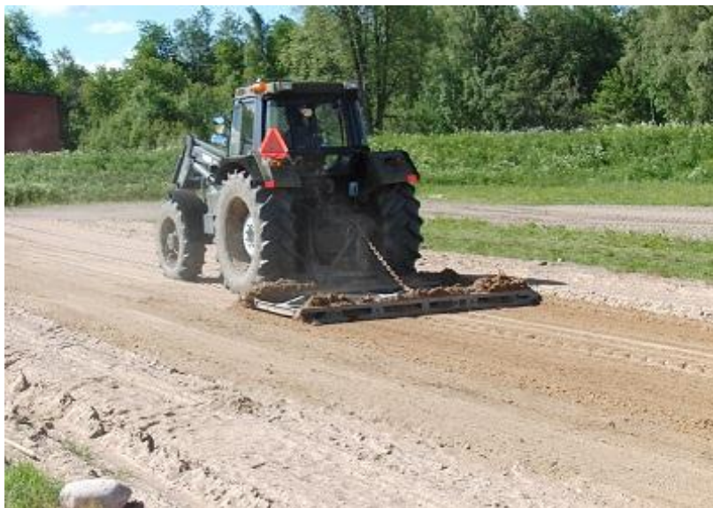
Figure 46. Step 2 – Running over the lane with a clod-crusher.
