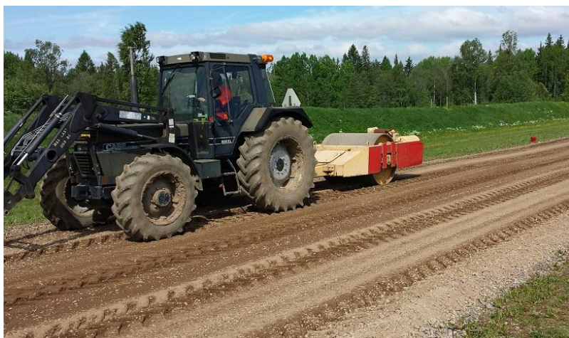
Figure 47. Step 3 – Compacting the lane
