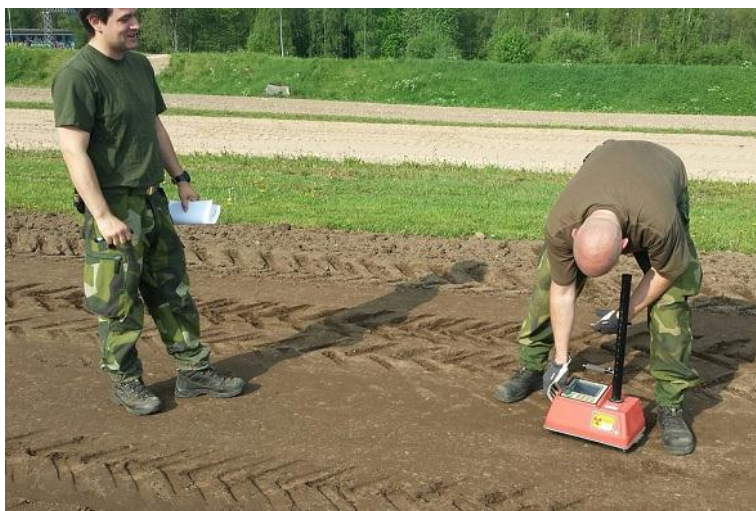
Figure 48. Step 4 - Measurement of compactness and moisture content.
