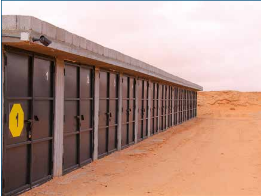
Figure 11 – Medium-walled Explosives Storehouse (ESH) 132)
