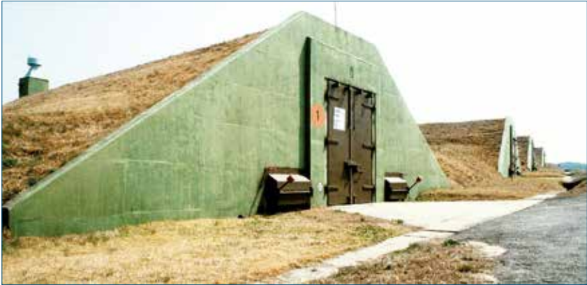
Figure 12 – Earth-covered magazine “igloo” type Explosives Storehouse 136)
