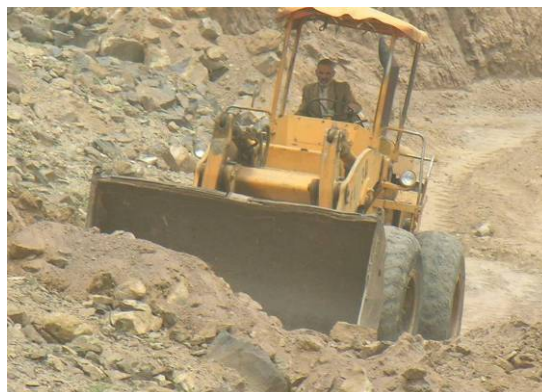
Building new terraces in demined land in Bait 'Oqab
