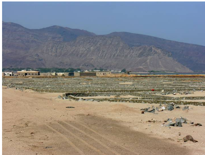
The original fishing village of Al-Farsi in Aden governorate has been surrounded by the foundations of 2,600 new houses to be built for the employees of the Aden Refinery Company at a cost of around US$11 million
