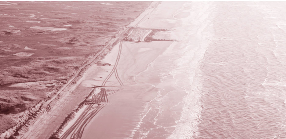
Beach areas which have been searched from surface to -75 cm with the top layer removed, ready to be searched from -75 to -150 cm
