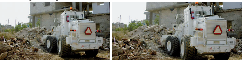
MSB Front-end loader moving rubble (Photo by Magnus Bengtsson)
