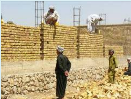
Building work is in progress
