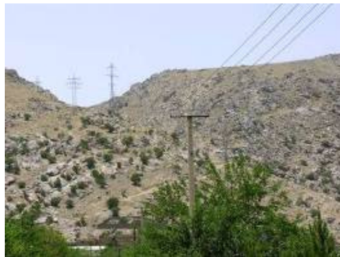
Clearance has allowed the construction of this high voltage electricity line
