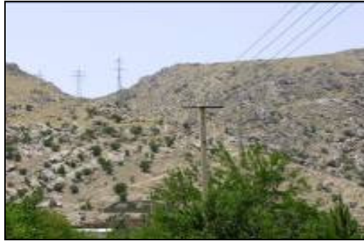
Photograph 6 – Power lines crossing cleared land
