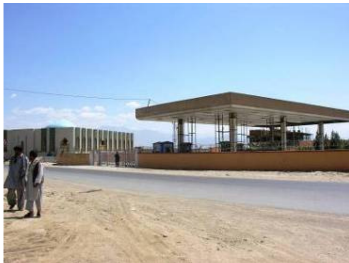
Filling station and mosque built on cleared land
