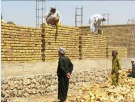
Building work is in progress
