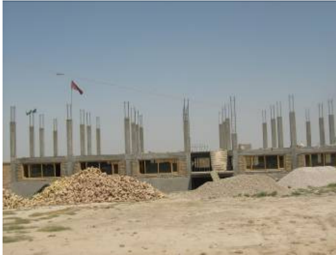
Construction near cleared areas
