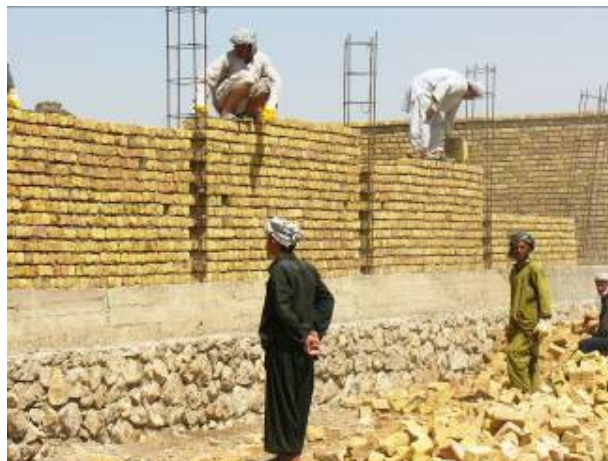
Construction of houses on the cleared area
