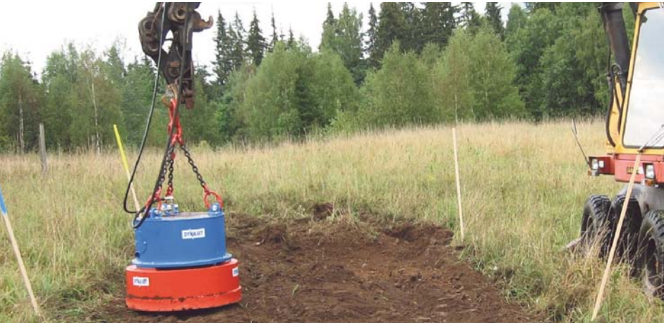
An electromagnet operated from an excavator
