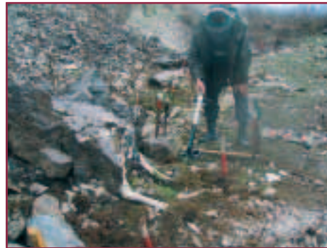
Fig. 3. A typical, obstacle-strewn manual demining lane on the southern bank of the Gumista river. Note the animal bones in foreground.
