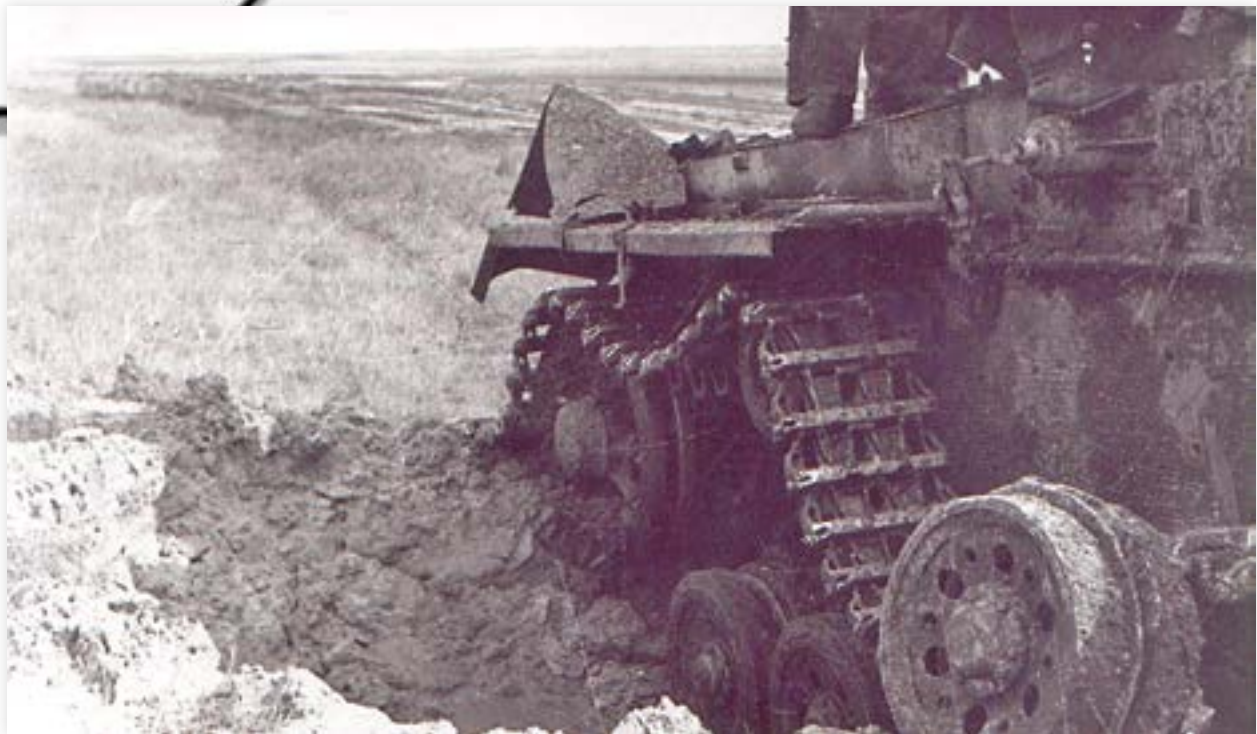
Image 21. Damage caused by an anti-tank mine on the track of a Panzer III during a “Test Run” of a minefield, Jutland, Denmark, summer 1945.
