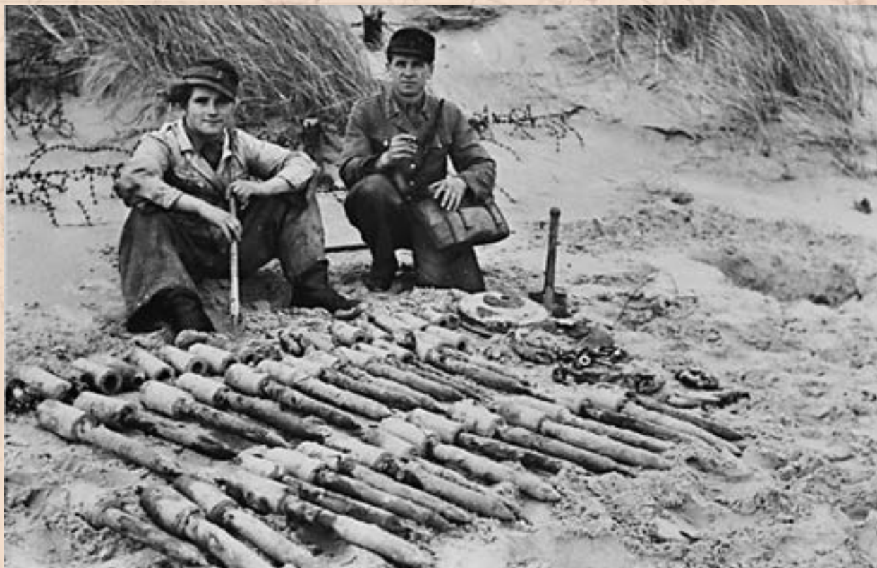
Image 7. Members of Minekommando Dänemark pose with a number of Stockmine 43s and three Tellermine 42s cleared from a nearby minefield, Jutland, Denmark, summer 1945. Image courtesy of Dan Mouritzsen - Silkeborg Bunkermuseum Denmark.
