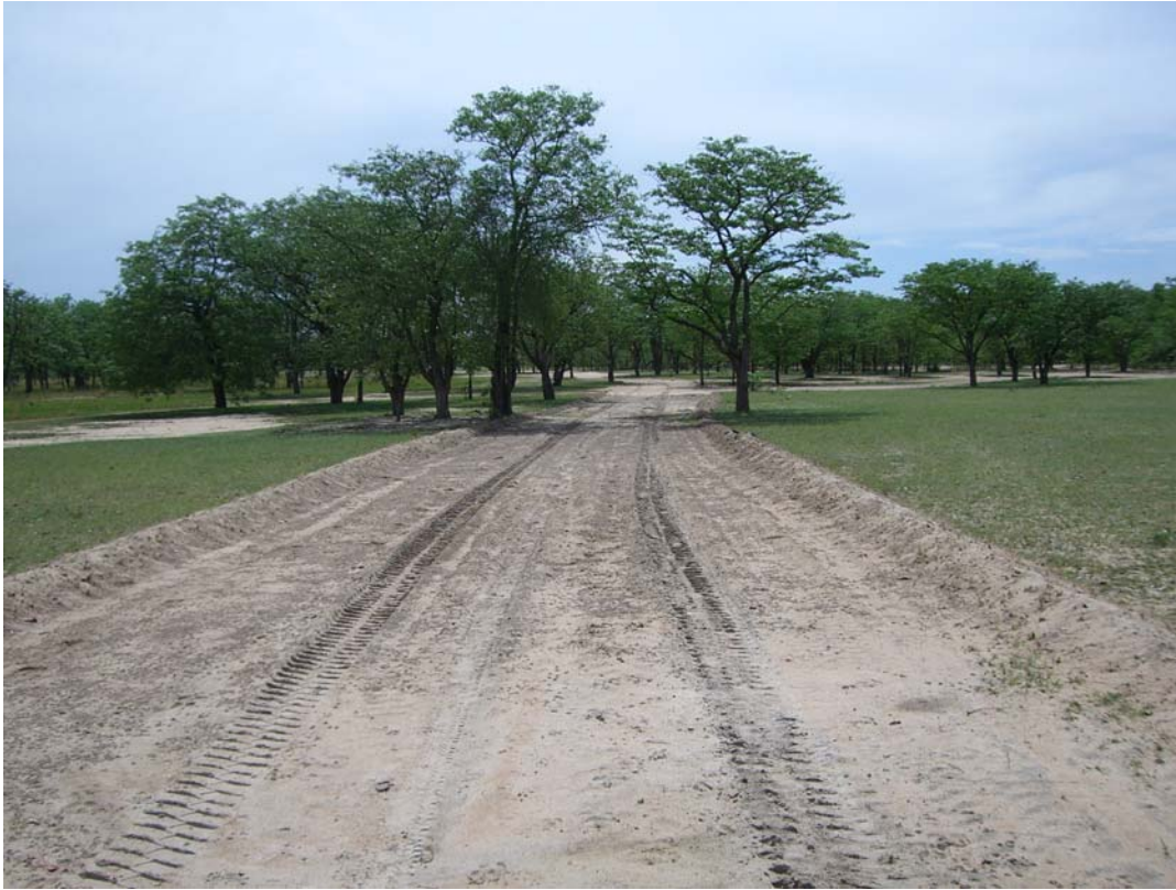
17. MgM road clearance in Angola.
